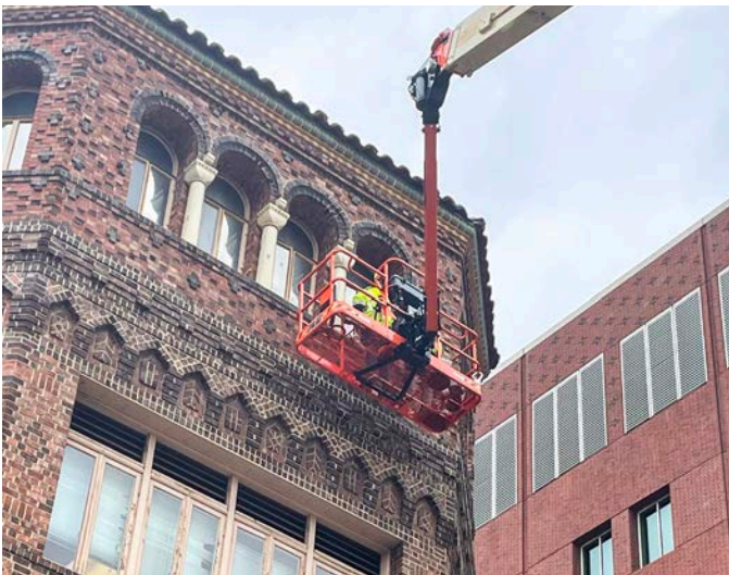
Routine Maintenance of Historic Campus Buildings
