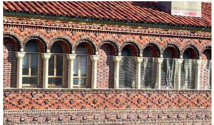
Protective Netting Installed on Historic Buildings
